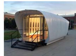
d) the AMIE demonstration structure printed by the Big Area Additive Manufacturing (BAAM) system. Image: courtesy of Oak Ridge National Laboratory, USA.
