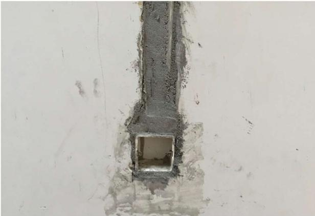
Fig.4. electrical services not integrated into the printing process. Courtesy of Wu et al. (2016).
