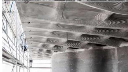
a) 3D printed formwork for a light weight ceiling of the Smart Slab project. Image: courtesy of ETH Zürich.
