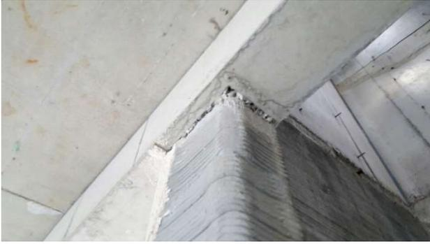
Fig.3. Unestablished joint system between structural member and extrusion-based 3DCP parts.
