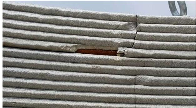
Fig.1. Building wall built by extrusion-based 3DCP technology shows defective tearing of concrete filament caused by cold joints. (Winsun).
