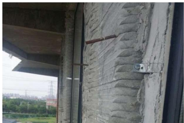
Fig.2. Awkward joint detail between 3D printed part and other building components.
